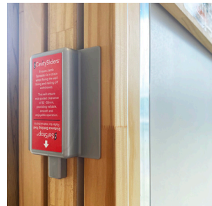
The supplied Jamb Spreader should be used during install.
